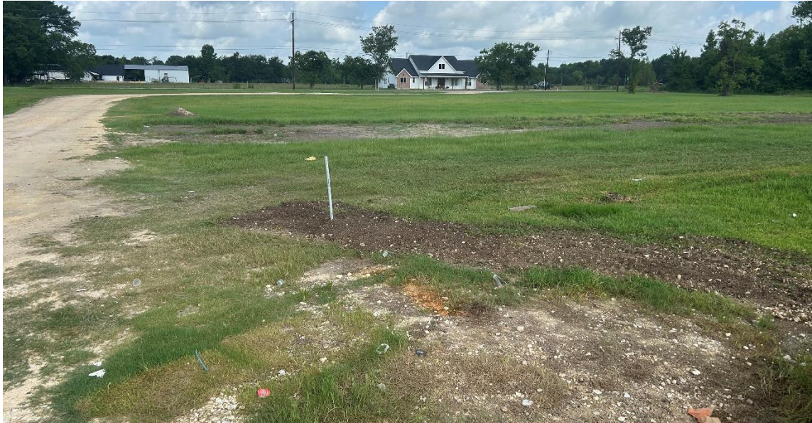
Sawmill Park (contractor trenching to property line for electric gates)
