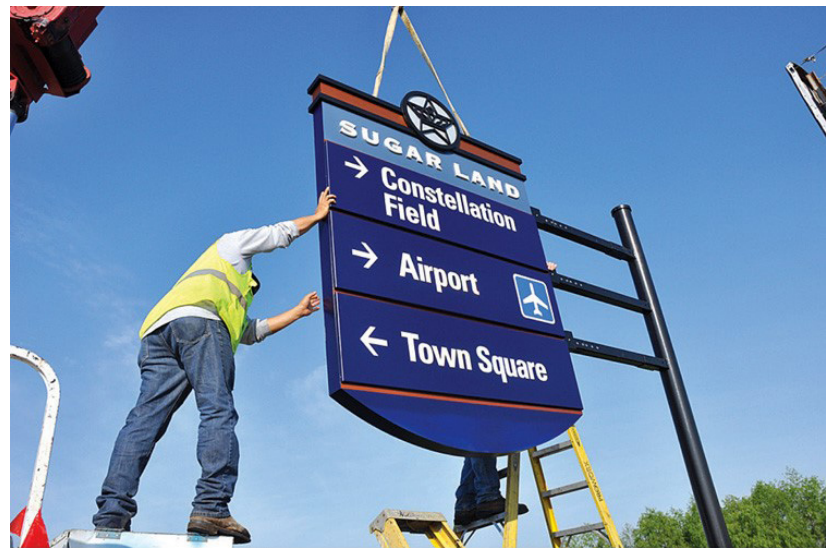
Precedent Example: Wayfinding in Sugar Land, TX
